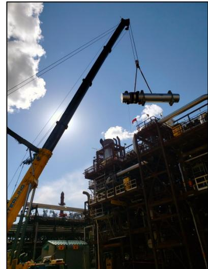
Sections of pipe are removed as repairs are underway to fix the stress cracks. (Photo credit: Sterling Crane)
