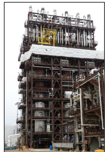
The new reactor burners will be installed inside this portion of the Gasifier to complete final testing.
